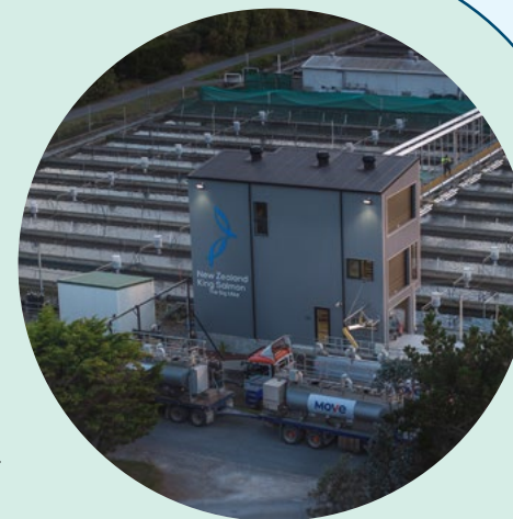
Image: The 'Big Mike' building at Tentburn.
