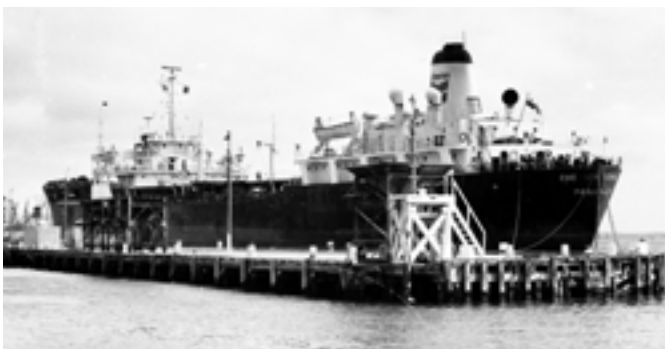
1975 Petroleum tanker Chevron Venice at the Town Wharf on 7 March, 1975.
