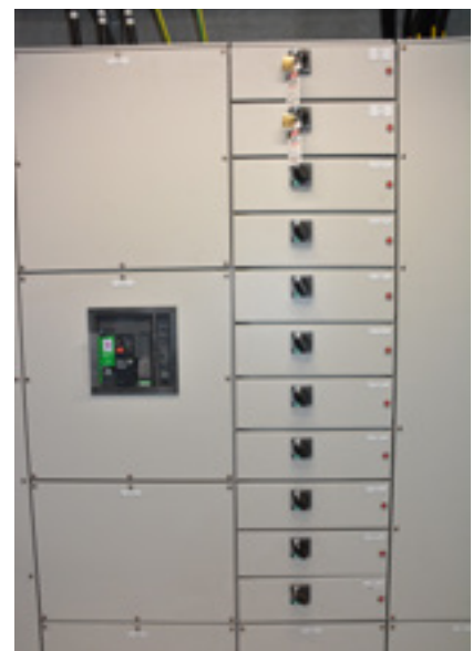
Substation B after the work was completed.
