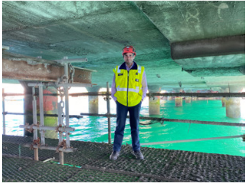
Site Engineer, Andrew Hill, under the access bridge.
