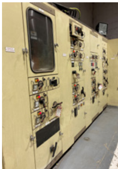
Substation B before the work was completed.
