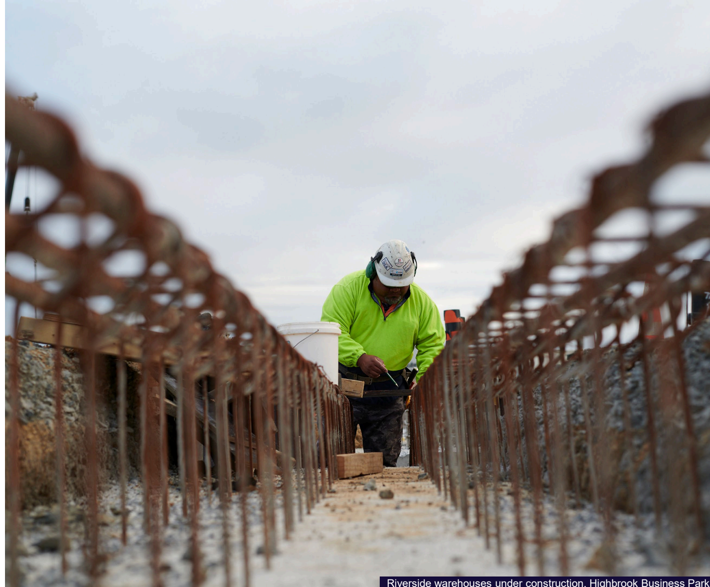
Riverside warehouses under construction, Highbrook Business Park
